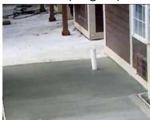
New Concrete for Stormwater Management
